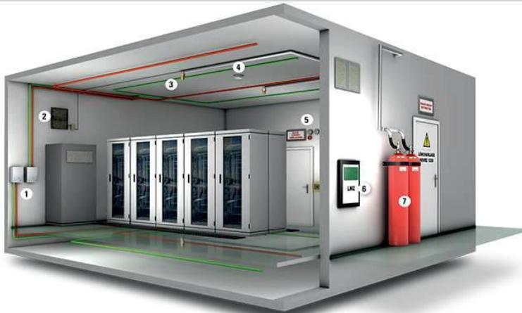
FK 5-1-12 fire extinguishing agent is a long life and sustainable solution in fire protection applications with special hazard classes. This second generation Halon alternative ensures high human safety, minimum environmental impact and provides superior extinguishing performance its Ozone Depletion Potential (ODP) equals to zero, has an Atmospheric life time of only five days and a Global Warming Potential (GWP) of 1.
